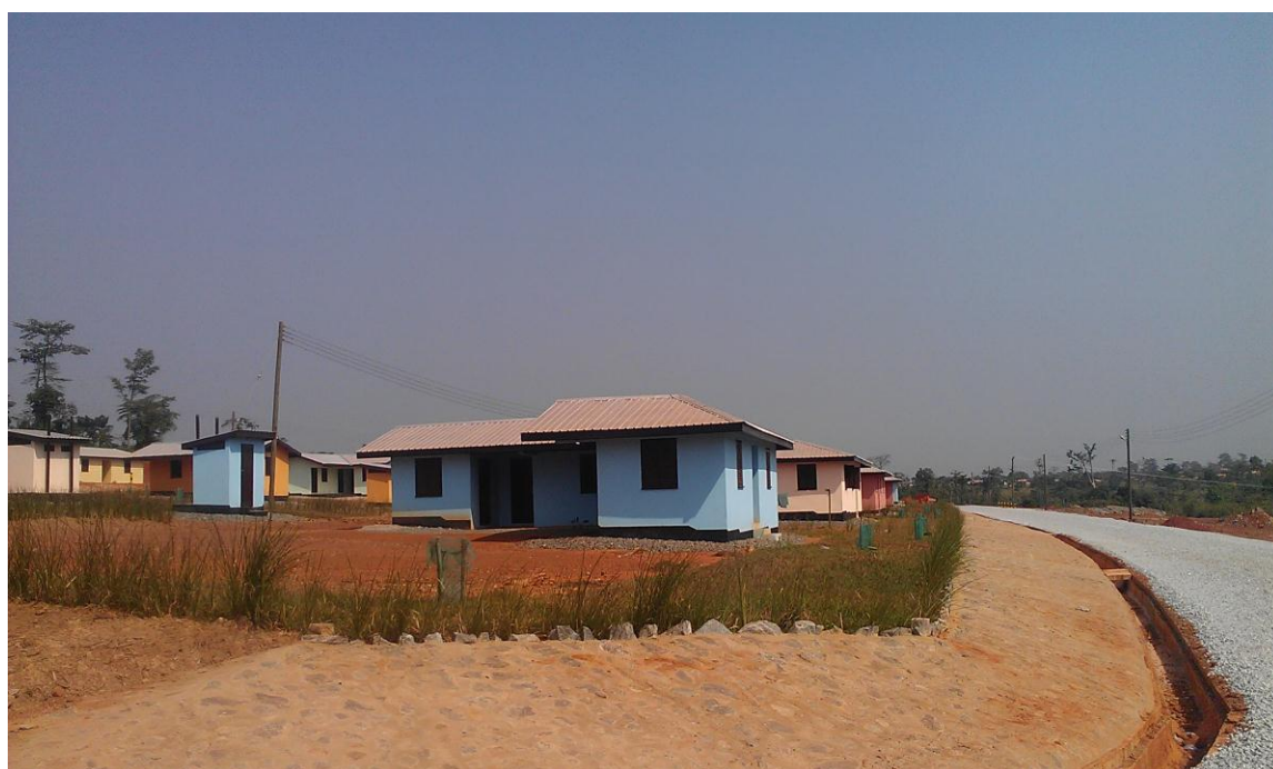
Figure 7-2. View of New Resettlement Site for Ahafo South Expansion PAPs (Kenyasi 1?)
